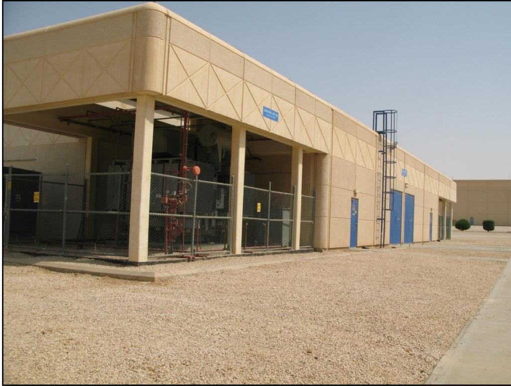
Picture 2: One of the Main Electric Power Distribution Substations
