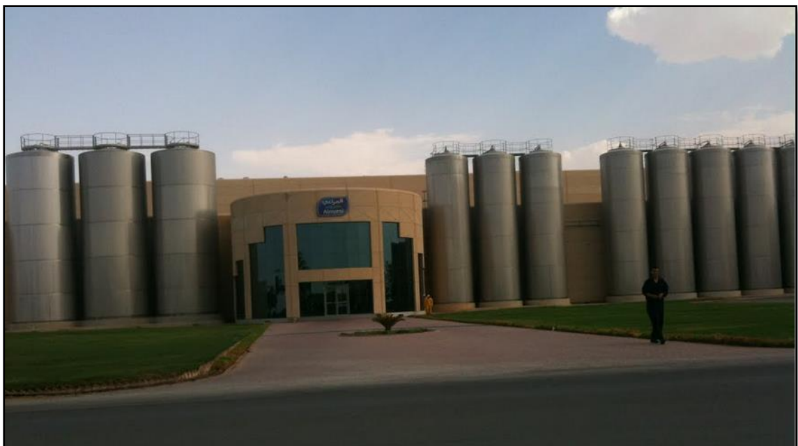
Picture 1: General plant view
