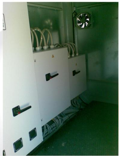
Picture 12: Interior of a Substation that contains LV Variable Antiresonance Harmonic Filters
