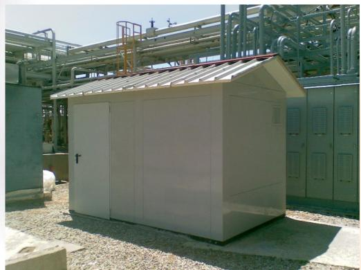
Picture 11: Low Voltage (LV) Variable Antiresonance Harmonic Filters installed into Substation due to special explosive environment
