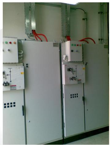
Picture 15: Conductor, Circuit Breaker and Control of the MV customized intervention for one of the Rectifiers.
