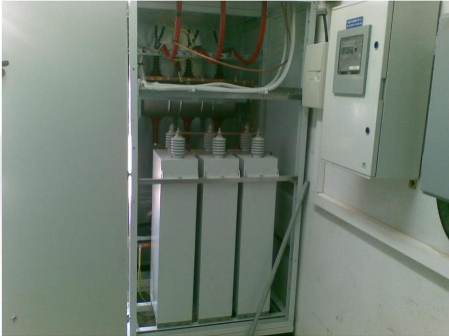
Picture 13: Inside view of the MV customized intervention for one of the Rectifiers.
