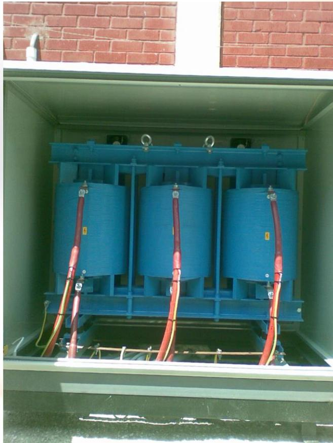
Picture 14: Special Harmonic Reactor of the MV customized intervention for one of the Rectifiers.
