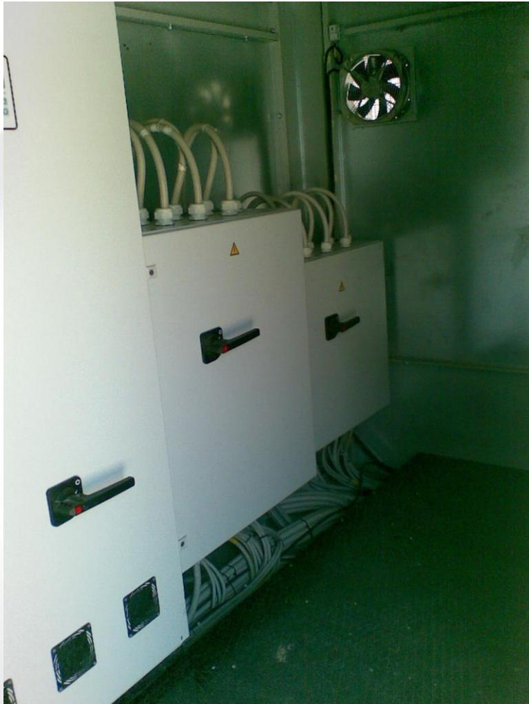
[Picture 12: Interior of a Substation that contains LV Variable Antiresonance Harmonic Filters](#)
