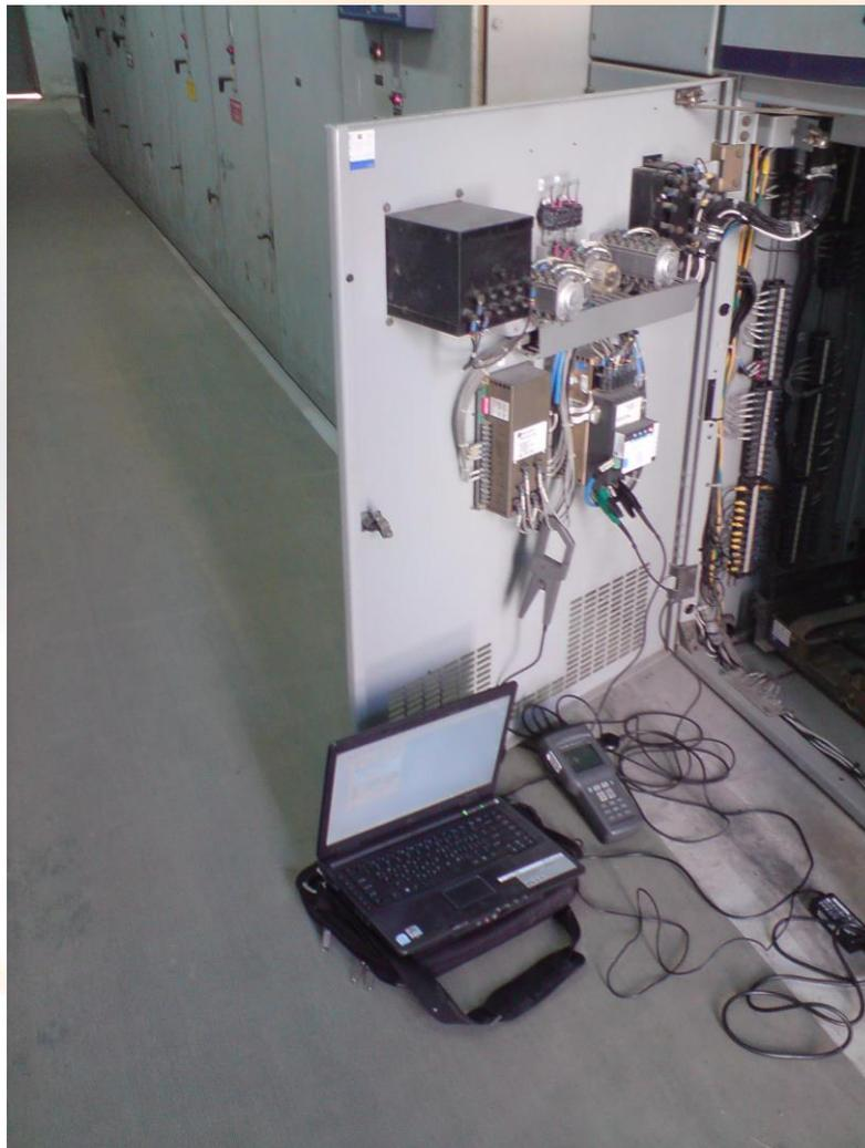
Picture 5: Laptops and Analyzers used for measurements and recordings
