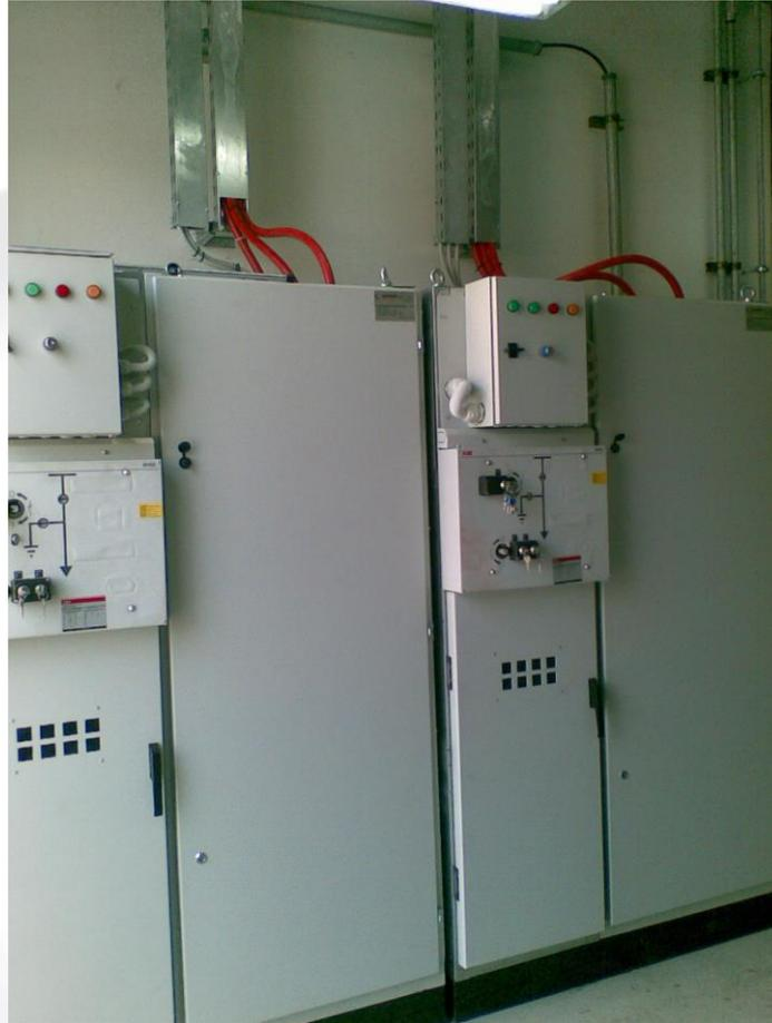
Picture 15: Conductor, Circuit Breaker and Control of the MV customized intervention for one of the Rectifiers.
